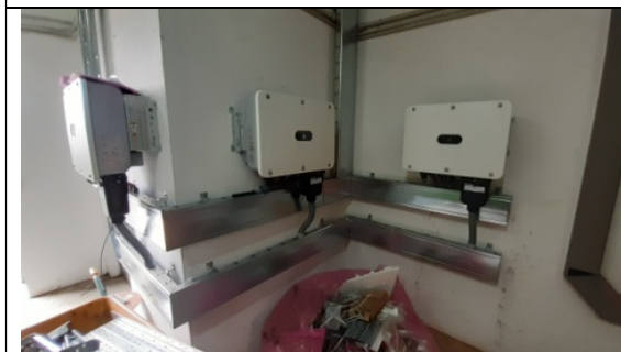
3 inversores Huawei SUN2000-30 KTL M3
